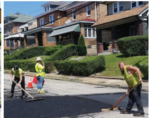
On August 24, Folino Construction installs speed humps on California Ave in response to a traffic calming study submitted to The Department of Mobility and Infrastructure by the BHCF in March of 2020. Jimmy Schropp runs a hand paver, Keith Cashmere moves asphalt to grade, Dave Blair operates a skid steer, and Tiffany McNany flags traffic.
