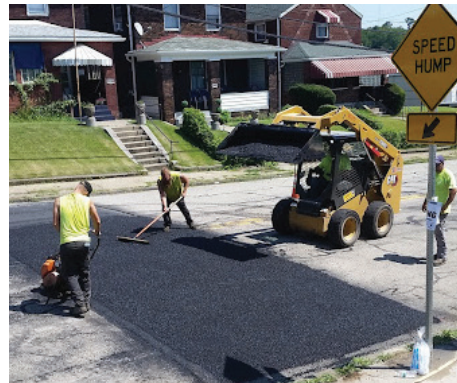
On August 24, Folino Construction installs speed humps on California Ave in response to a traffic calming study submitted to The Department of Mobility and Infrastructure by the BHCF in March of 2020. Jimmy Schropp runs a hand paver, Keith Cashmere moves asphalt to grade, Dave Blair operates a skid steer, and Tiffany McNany flags traffic.
