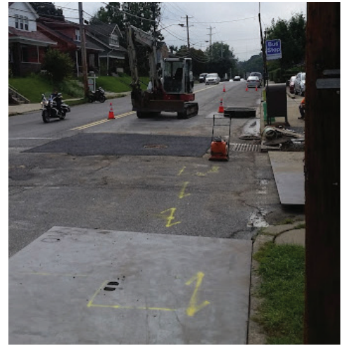
Subcontractors hired by PWSA complete repairs to a 15-inch terra cotta sewer line that created a sink hole at California Ave and Chellis St.
