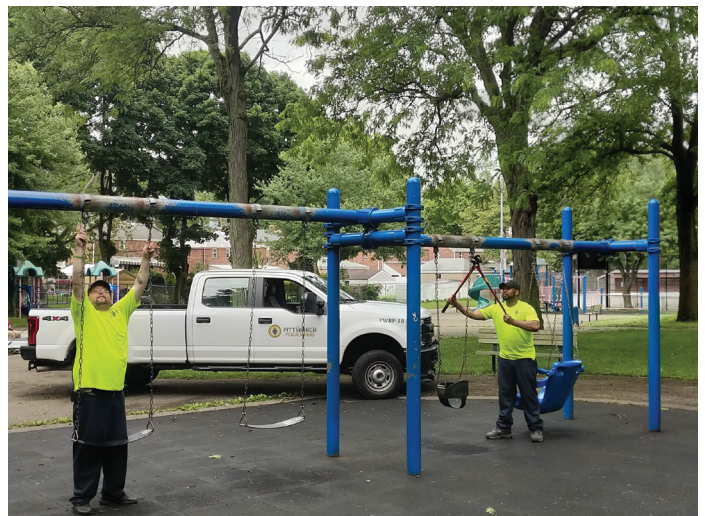
Pittsburgh Public Works Parks Division employee Jeff hangs a swing as Roosavonta uses a crimp tool to secure chains at Marmaduke Park when City parks reopened on June 15, 2020.
